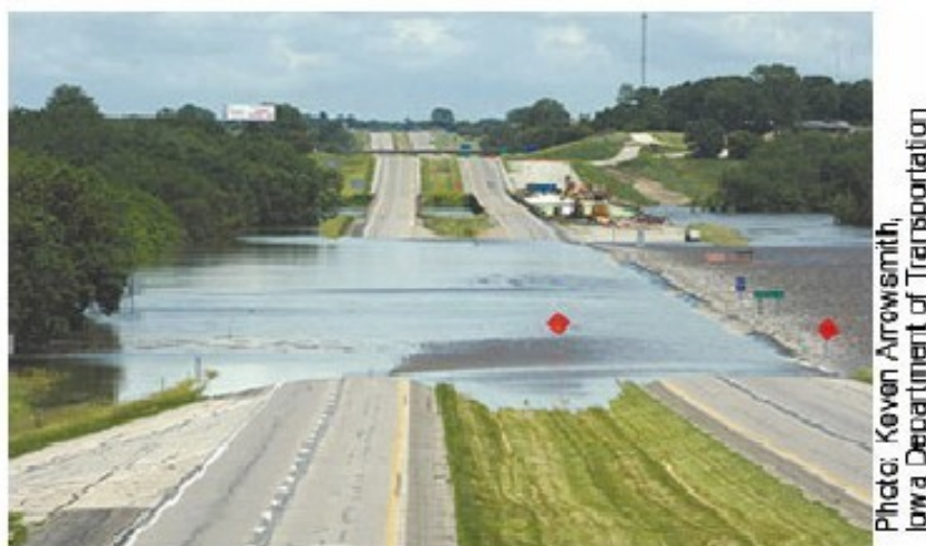
Figure 2.4 Submerged-flow of Cedar River bridge on I-80 in Iowa in June 2008
